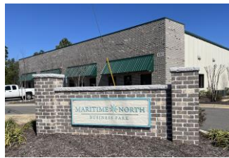
Maritime North Business Park 4270-4320 US Hwy 421 North Wilmington, North Carolina Purchase Price: $ 18,125,000 Type: Flex Size: 138k square feet
